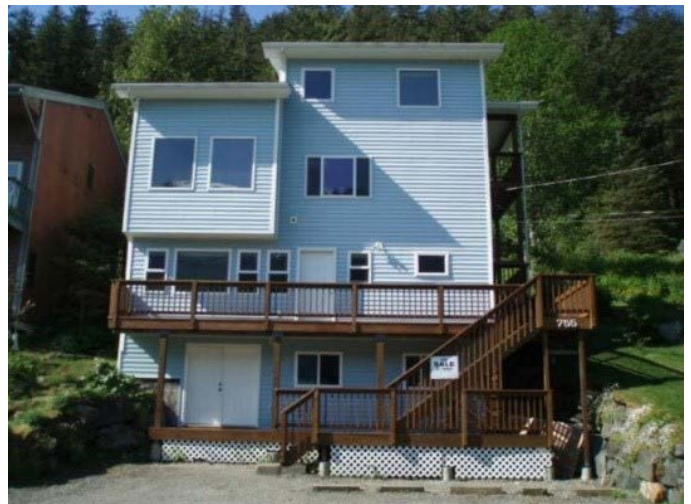
Attached ADU Added to the Basement of a Juneau Home Through the ADUG Program
