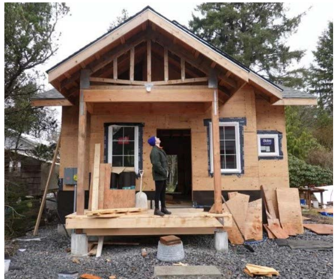
31-year-old Sitka resident Adrienne Wilber standing before her partially constructed ADU built on the corner of her parent's lot
