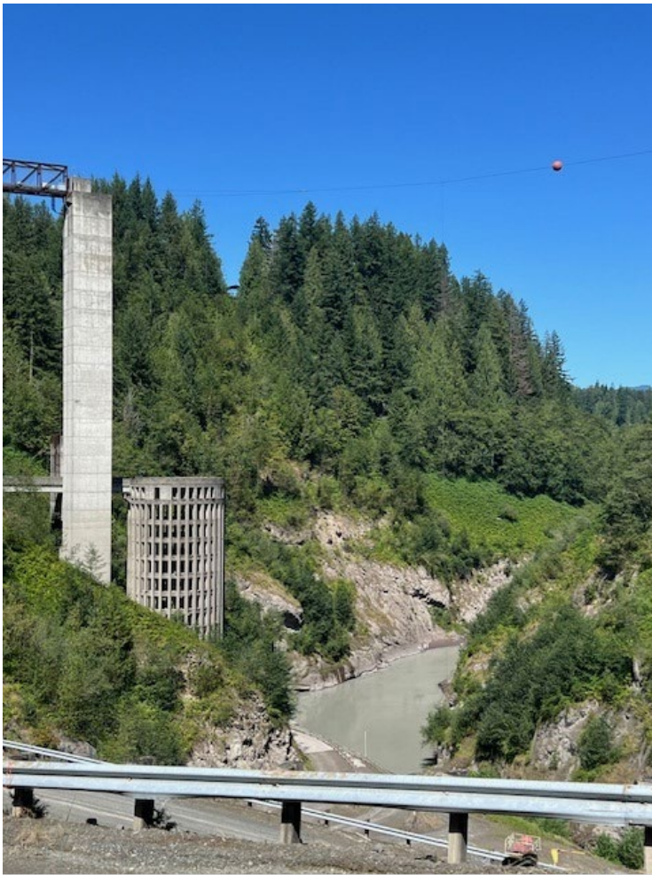
This is the honeycomb water intake and the tall square air vent for the tunnels. The water level is drained down very low. It is normally up to the rock ledge in the picture – sometimes over the green treeless area!
