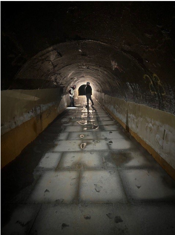
Mud Mountain Tunnel with granite block floor
