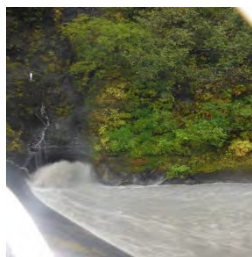
Lowell Creek Tunnel: Entrance
