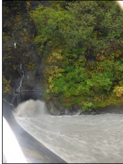
Lowell Diversion Tunnel-Upper Entrance
