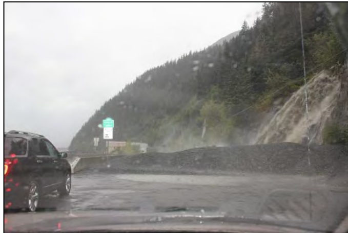
Lowell Creek Tunnel Debris Laden Outfall
