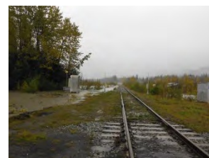
RR at Nash Rd-Acts as Levee
