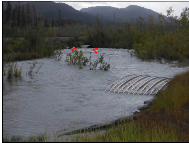
Figure 5-6 Undersized Culverts, Nash and Salmon Creek Roads
