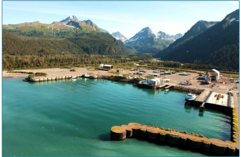
Figure 3: Existing SMIC Maritime Facilities
