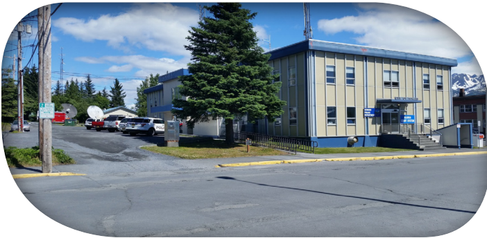
Figure 15 - City of Seward Police Station
